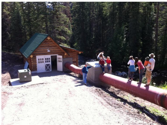
Figure 5: Humphreys Hydro Powerhouse
