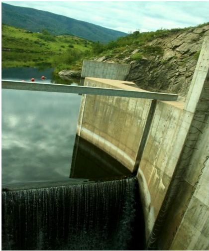
Figure 6: Lake Catamount Spillway
