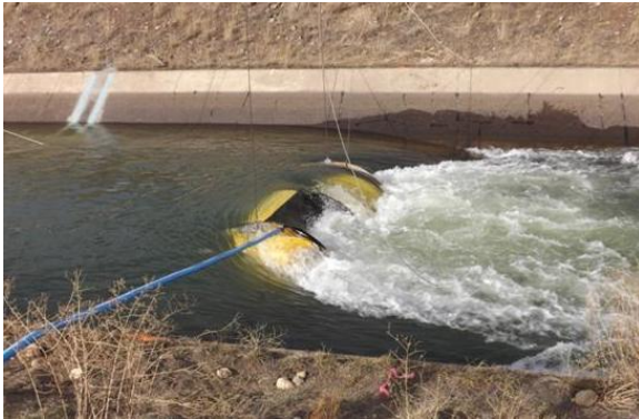
Figure 12:Hydrovolts – Roza Canal
