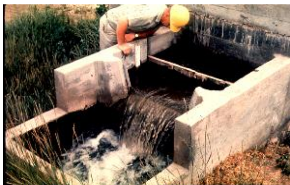
Figure 19: Cipoletti Weir
