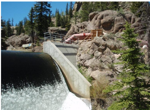
Figure 6: Humphreys Hydro Siphon Intake (Upper Right)
